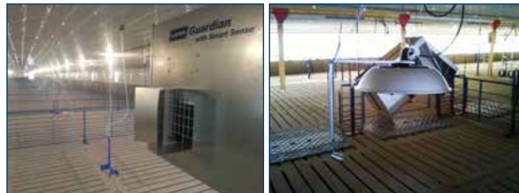
Works with a wide range of house controls that offer a 0-10 volt signal.
